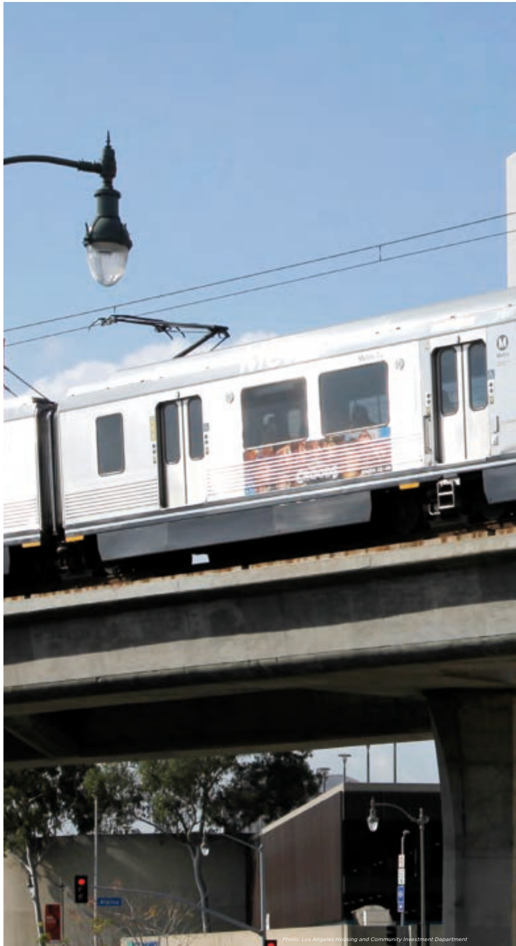
Photo: Los Angeles Housing and Community Investment Department
